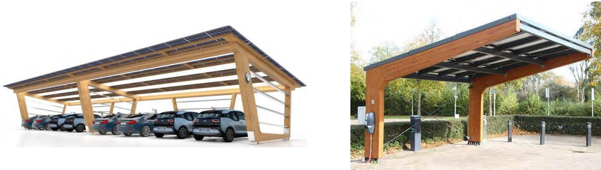
Figure 16: Examples of Solar PV in car parks
